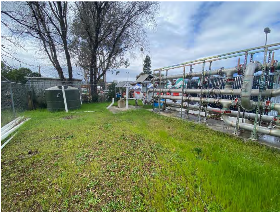
County Building Well
